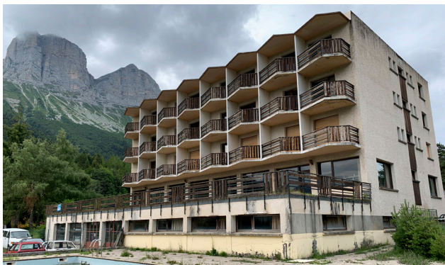
Fig.002. Existing building the Team AuRA is working on
